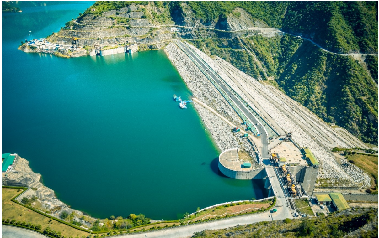
“The Giant top view of India’s Highest Earthen Dam - Tehri Dam, Uttarakhand”
