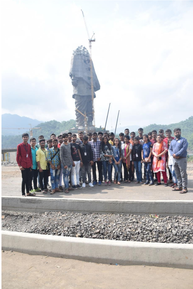
“Work has been completed upto full body”
