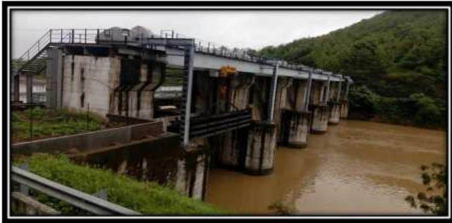
Canal Head regulator, Narmada
