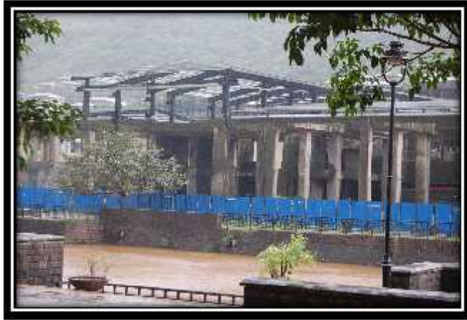
Rcc & Steel Structure, Lavasa
